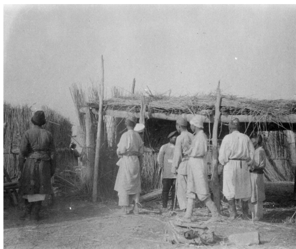
Fig. 9 Loptuq men constructing a satma , a new reed hut with wooden structure at the hamlet Dilpar in 1934 (Photo David Hummel)
